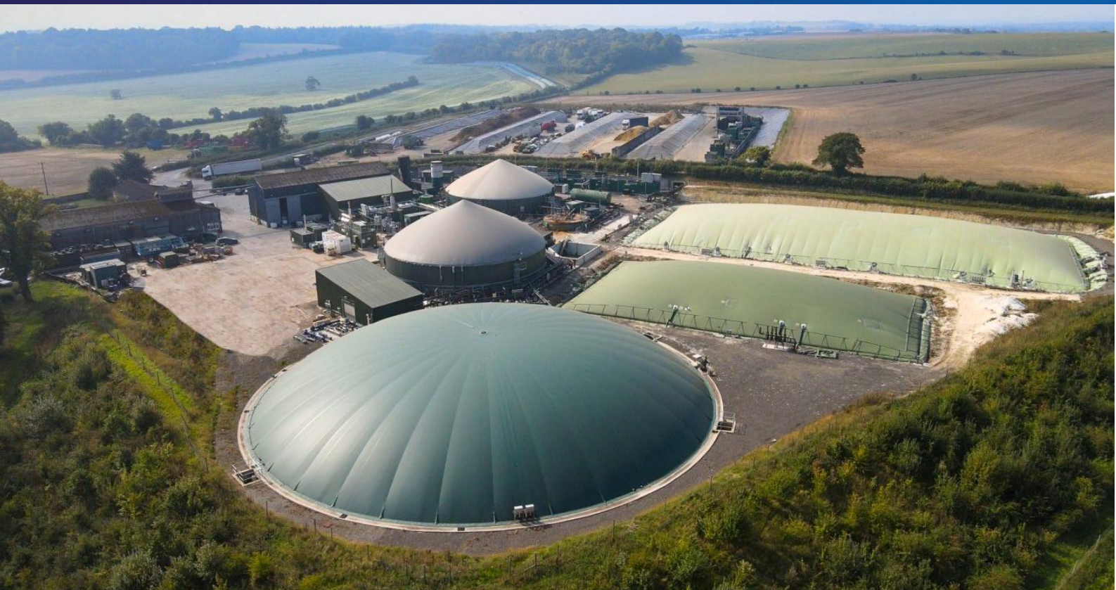
Figure 1 Overview of Apsley Farms biomethane plant
