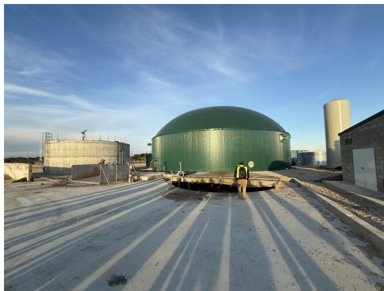
Figure 10: Alcarràs Biomethane Plant, Catalonia, Spain, site visit
